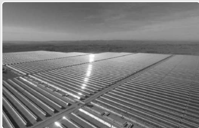
solar panel farm in Ouarzazate
